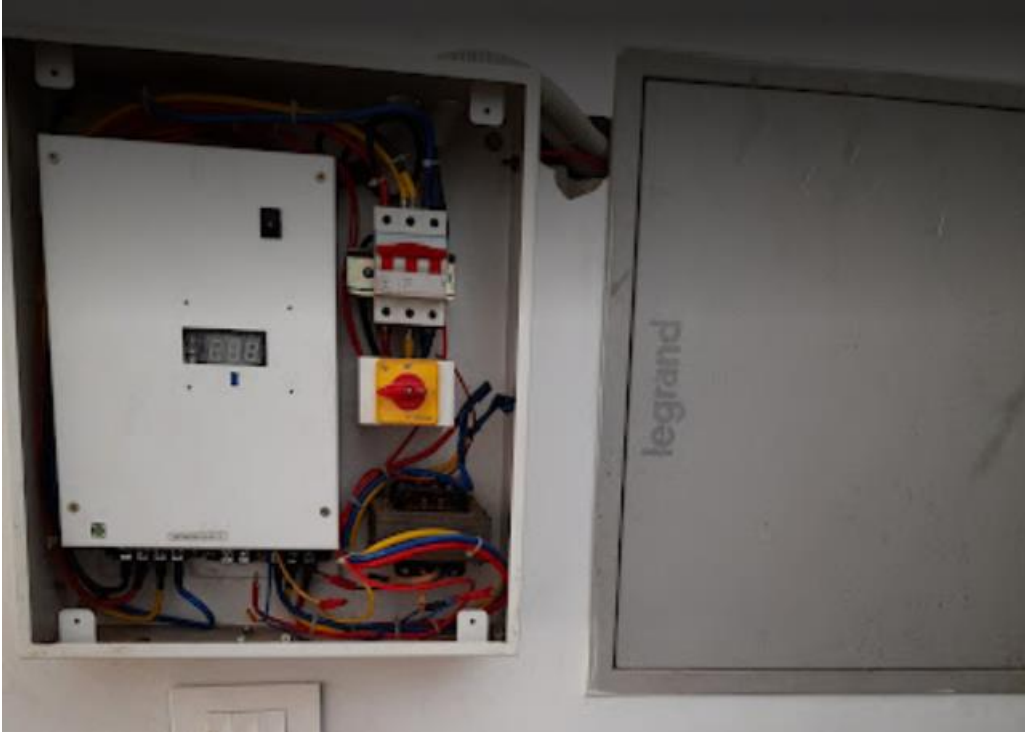
Traditional Protector(Lot wall work and Limited level of protection)
