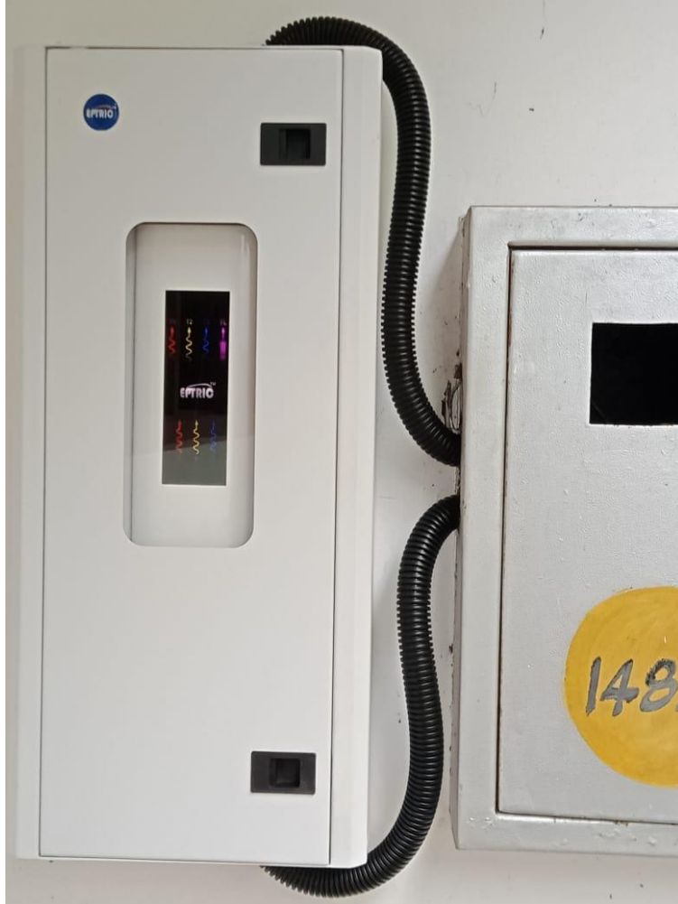
Distribution box with out Selector switch case needs external fix enclosure
