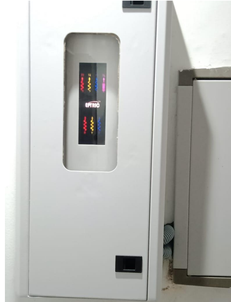
Distribution box with out Selector switch case needs external fix enclosure
