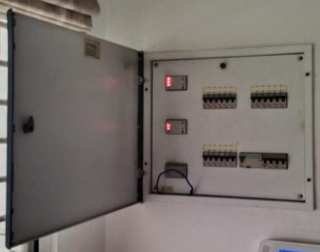
Model : Crabtree Phase Selector DB
