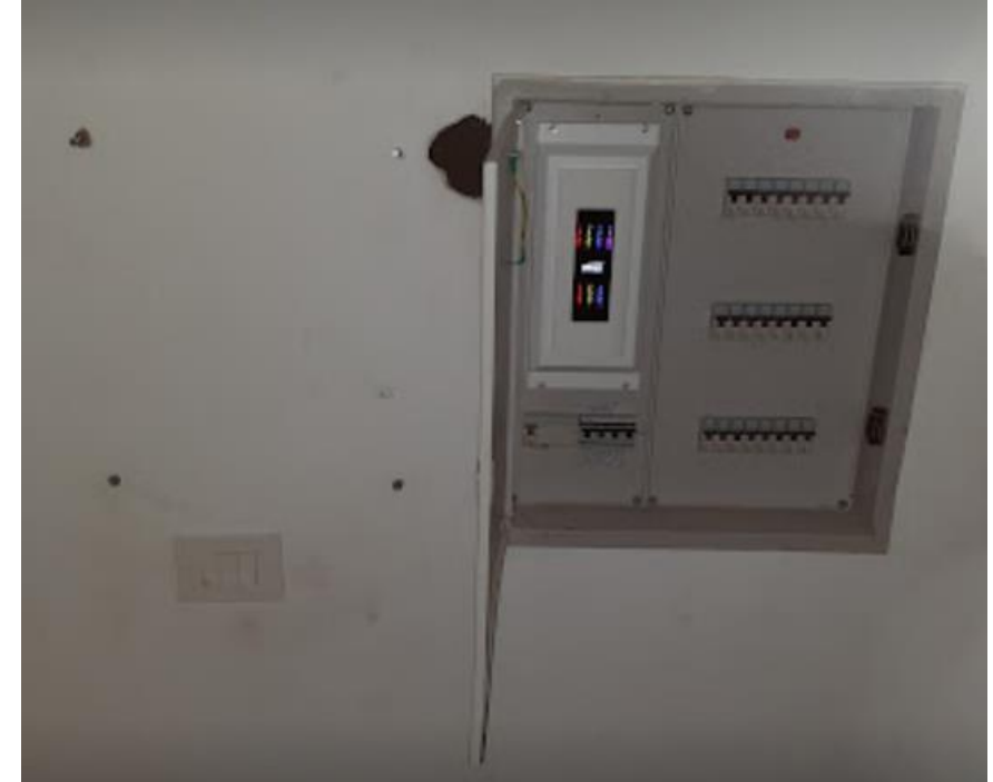
APS integrated to exiting DB with out wall alteration and comprehensive protection
